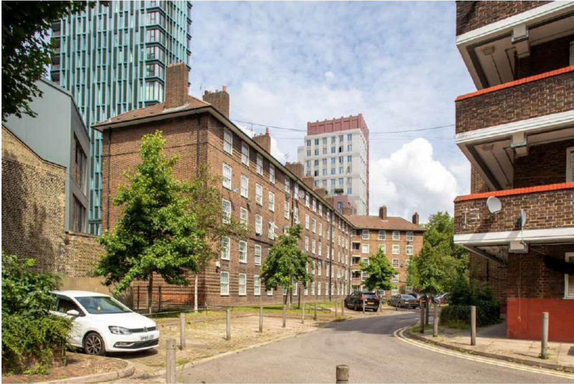
View 2 (Stephenson House to the East of the Railway Viaduct)
